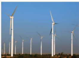
The first wind-power generation project established by Chinese companies in Karachi, Pakistan.
