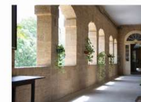
The building has semi-circular openings at the ground floor and segmented ones on the first floor.
